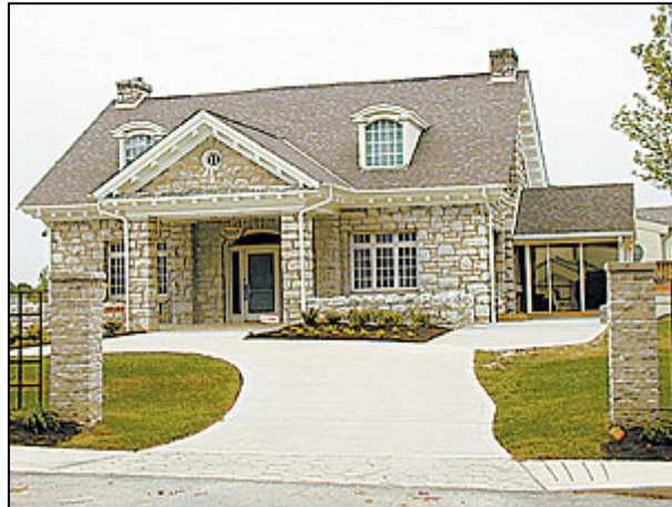
Best Restoration - 12102 Old Big Bend
